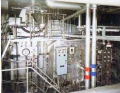
HDN-25S 25t/h x 60kg/cm 2 G x 425 degree C
